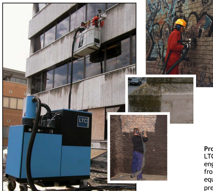
Removing dirt, coatings & graffiti from buildings
